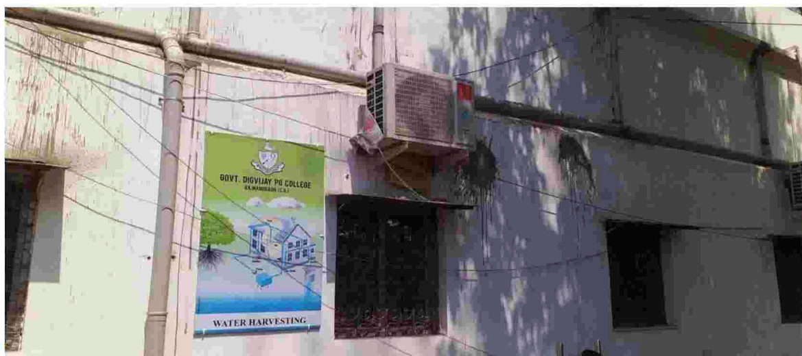
Fig: The installation of Rain water Harvesting System is adding more to the already sufficient ground water level.
